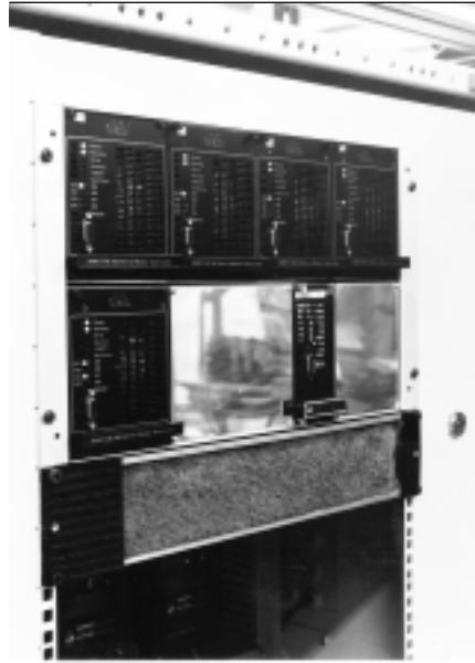
JVL and Systec Controllers mounted in a 19" rack in the control station.
